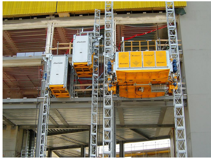
Higher capacity material Hoist model available in double mast
