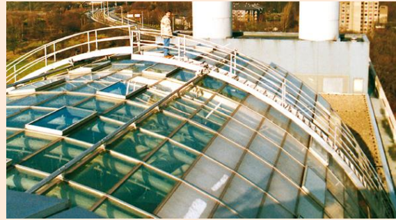
Gantry cradle over wide area glass roof
