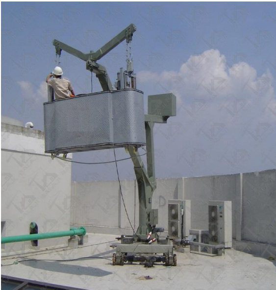
Cradle parks on the roof terrace after use
