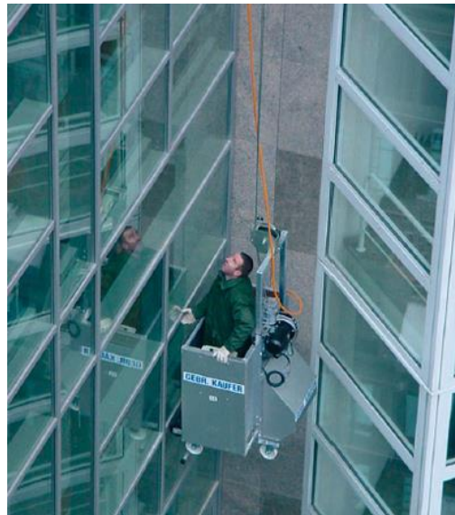
Solo cradle with suspended access system
