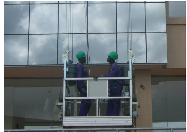
2-man cradle with suspended or monorail systems
