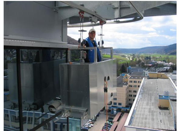
Monorail system with Cradle on the external facade
