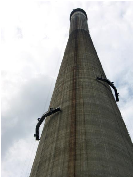
Suspended Access system - wide platform
